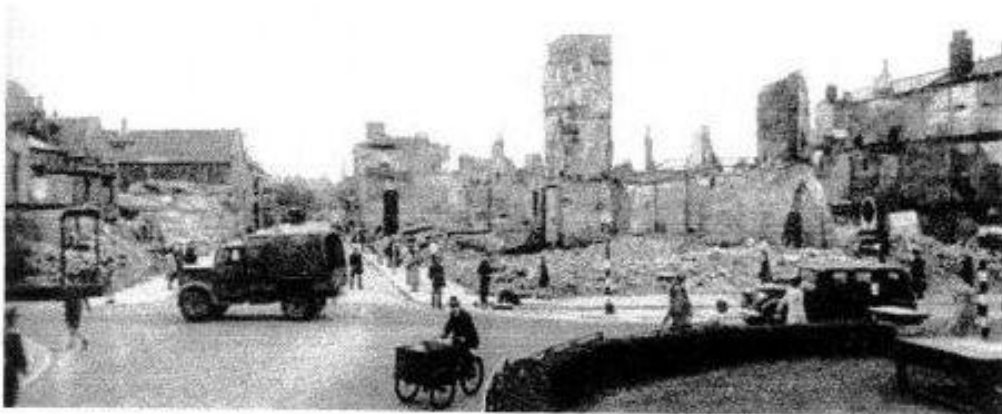
Bomb damage at Weston-super-Mare.
